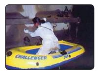
Visual examination and U.T.M. gauging of ballast tanks carried out during ballast voyage by the following ways:
